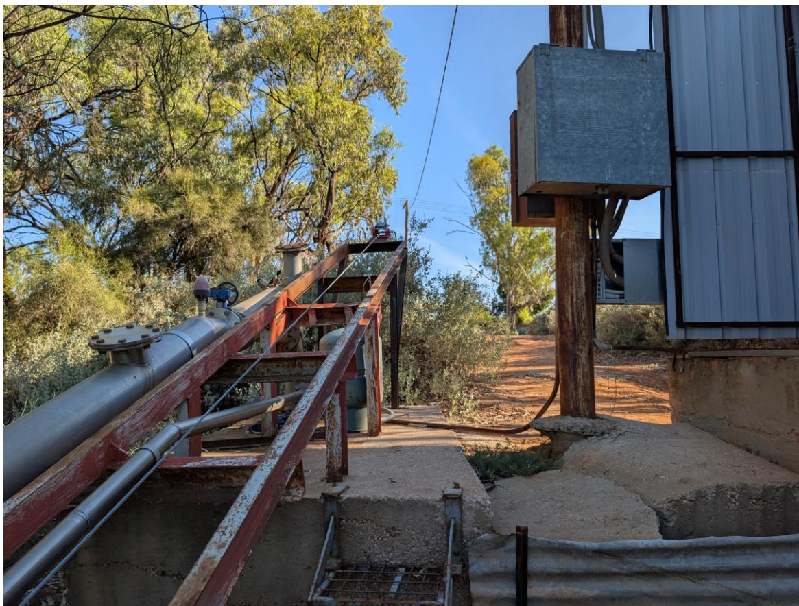
Figure 10: The existing structure to be removed includes old concrete footings. Measures to ensure no debris rolls downslope to the river.
